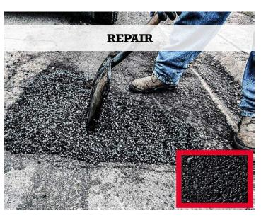
**Repair** is an all-weather patching compound used to keep shipping and loading areas, parking lots, drives, and walks in safe repair all year round.
