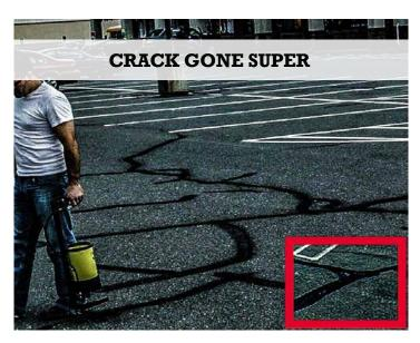
Crack Gone Super seals cracks where structures meet sidewalks and/or driveways. It produces a tough, flexible membrane that reduces water intrusion.
