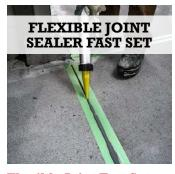
Flexible Joint Fast Set is a 100% solids polymer dual cartridge system designed to repair cracks and damaged expansion joints.
