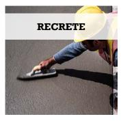
Recrete is a fast-setting mortar mix resurfacing and patching material for concrete, wood, and metal surfaces.
